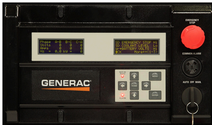
Digital H Control Panel—Dual 4x20 Display
